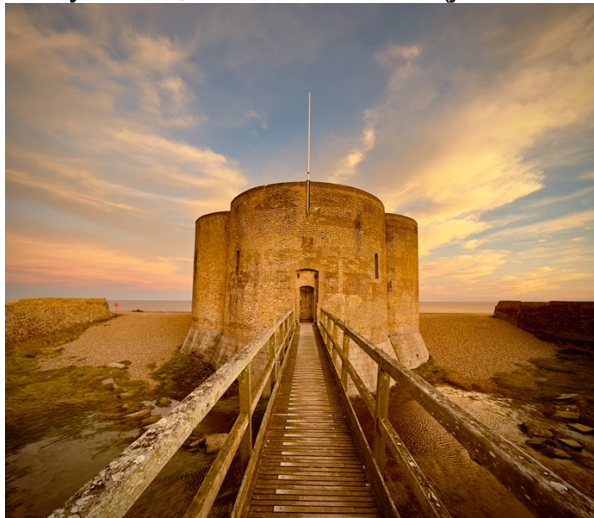
Aldeburgh Martello Tower © David Tolley
